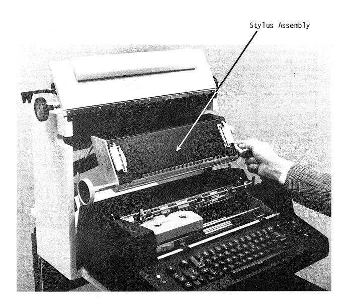
Figure 3. Braille Embosser Showing Stylus Assembly
